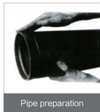
Lubricate gasket
