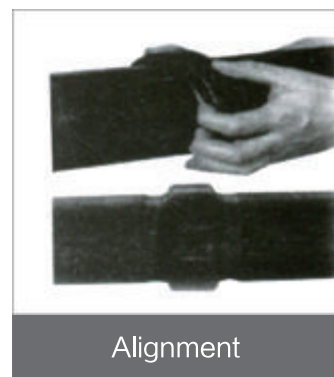
Gasket installation
